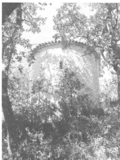
Elévation est, chevet. Phot. Julie Vidal IVR93_20220601384NUC1A
